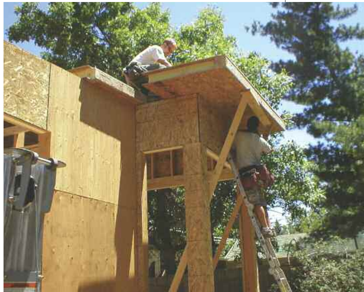
Energy-saving structural insulated panels (SIPs) being installed as the roof of a residential addition in Boulder, Colorado.
